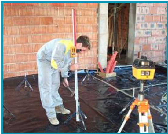
Using a laser level
