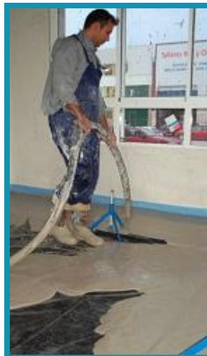
Placing Screed Gylvon
