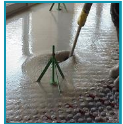
Levelling with tripods
